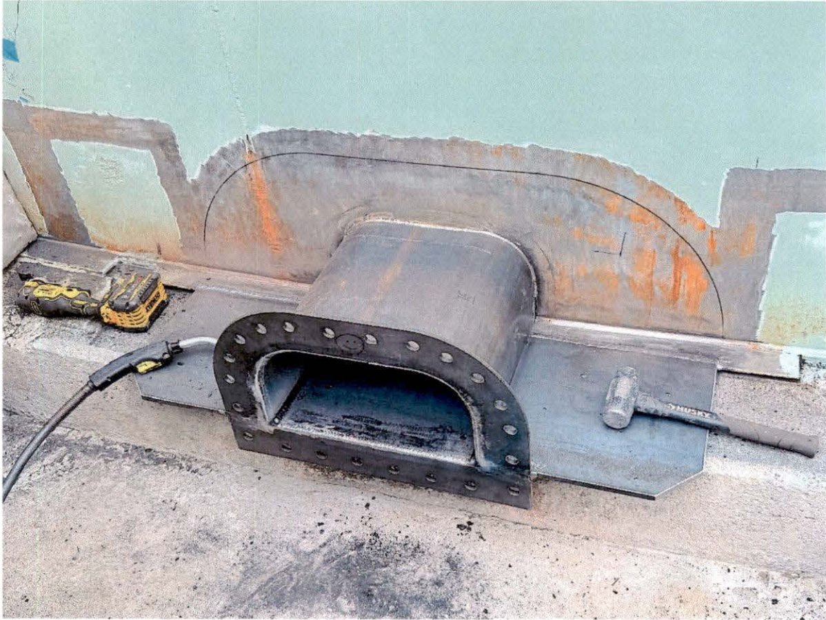
May 7, 2026 – Flush cleanout installation
