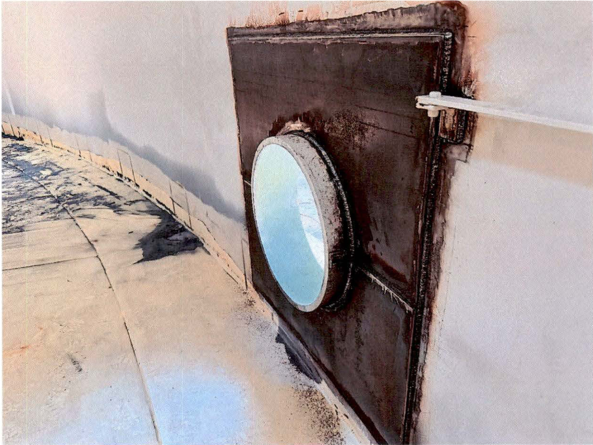
May 14, 2026 – Shell manway strengthening
