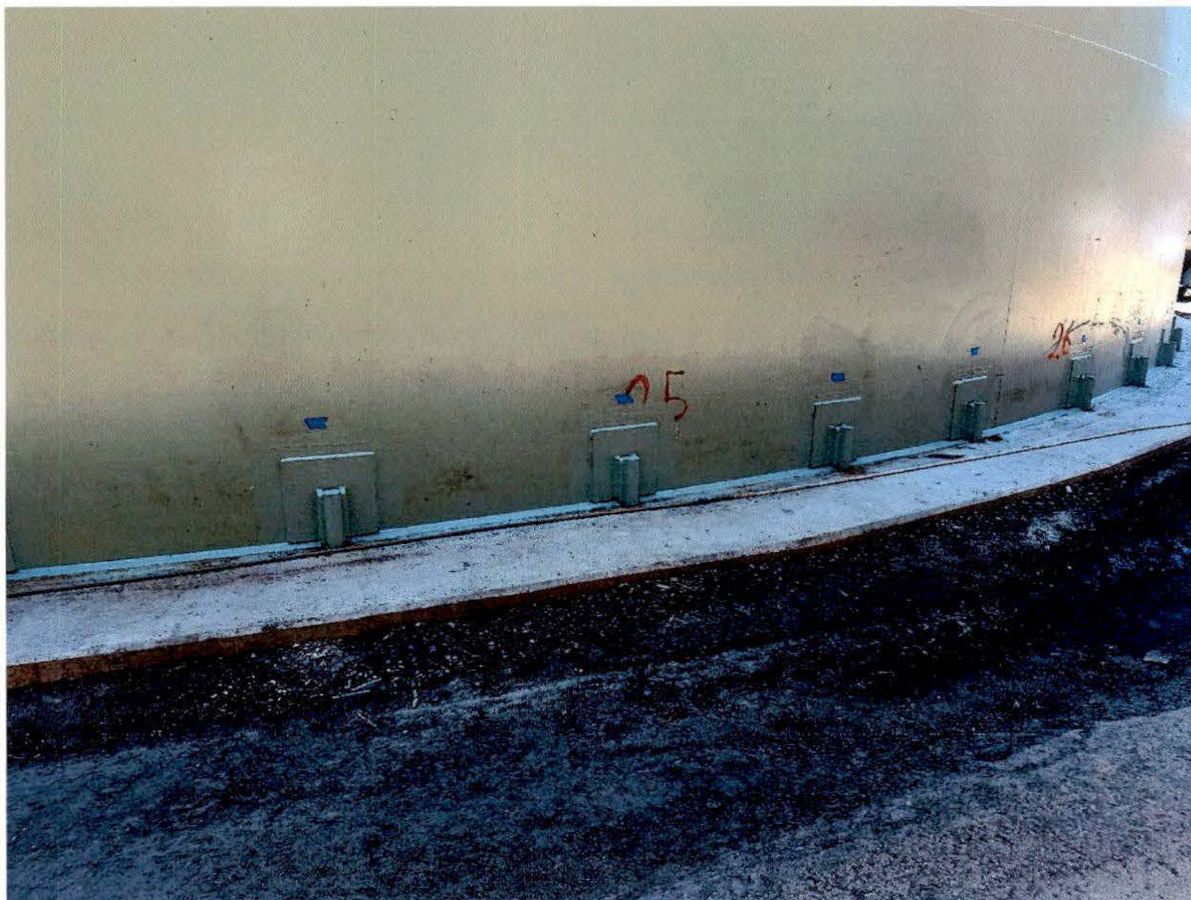
May 27, 2026 – Finished anchor chair installation & coating
