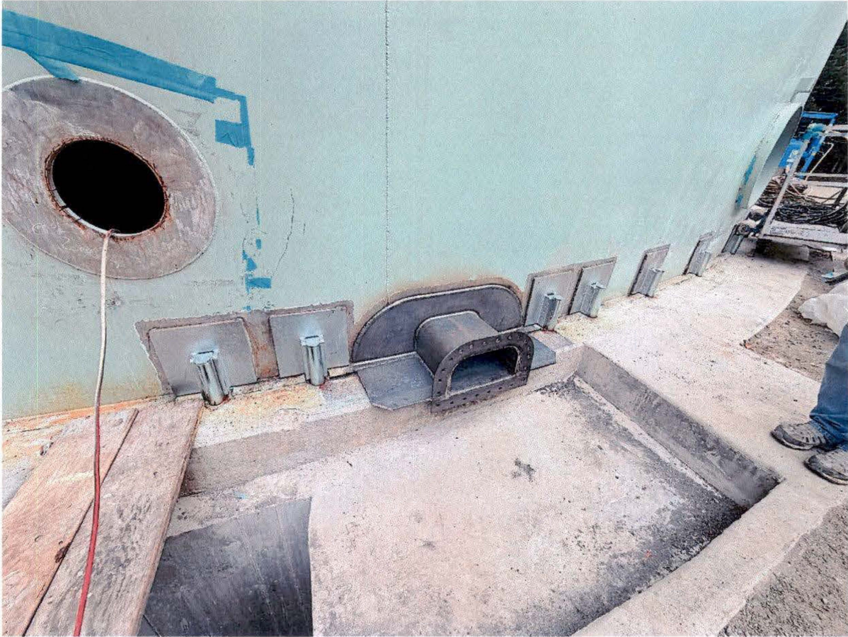
May 8, 2026 – View of new drainage basin at overflow/flush cleanout.
